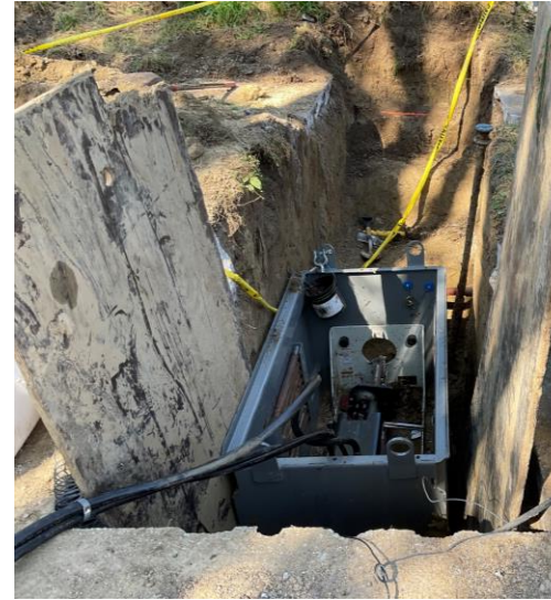
Pit Bore Setup
