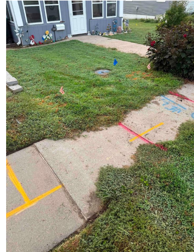
Meter Pit in Front Yard -Will be abandoned.
