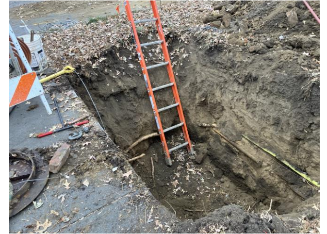
Typical Excavation at Stop Box
