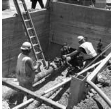
With telescoping spreaders and end panels pinned 1' up in corner posts, allowing utility to run through
