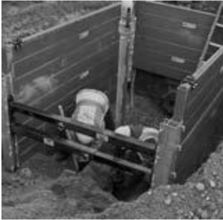
With telescoping spreaders and removed bottom panel
