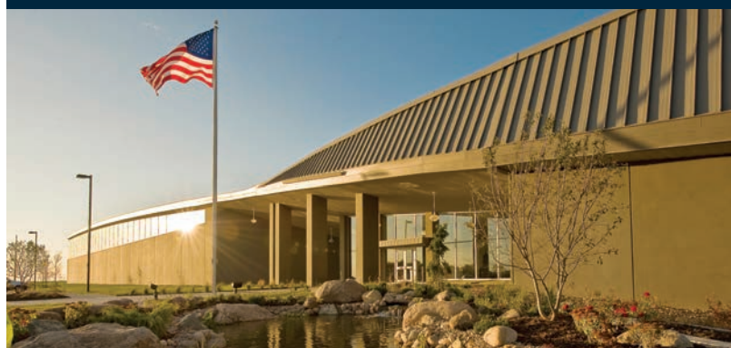
Platte West Water Treatment Plant
