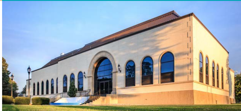
Florence Water Treatment Plant
