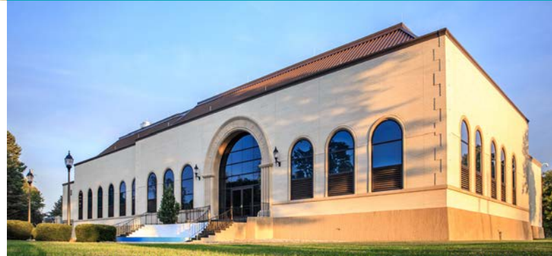
Florence Water Treatment Plant
