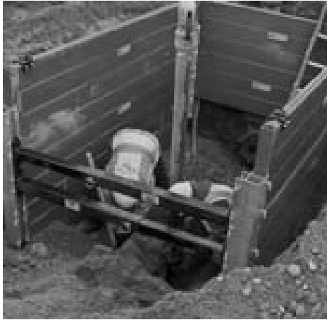
With telescoping spreaders and removed bottom panel
