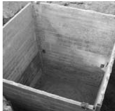
Stacked BUILD-A-BOX™ Modular Trench Shield System
