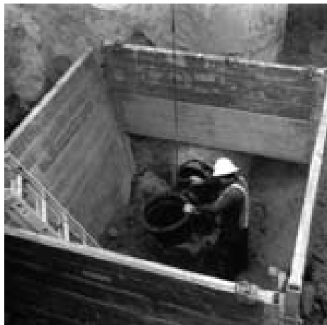
With sectional corner posts and removed bottom panel
