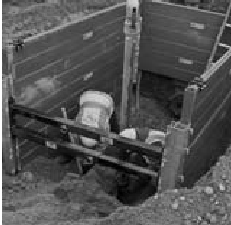
With telescoping spreaders and removed bottom panel
