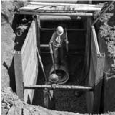
With telescoping spreaders and full length corner posts
