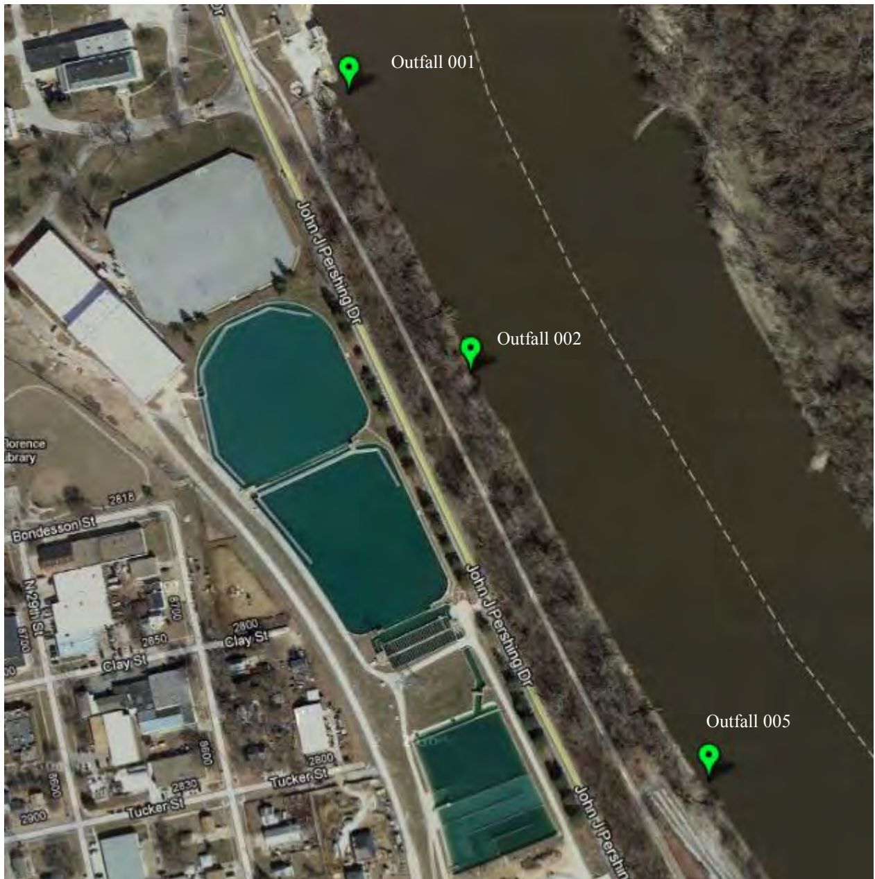
Figure 1. Location of Outfalls 001, 002, and 005 at the Florence PWTP (scale – 1”=400’)
