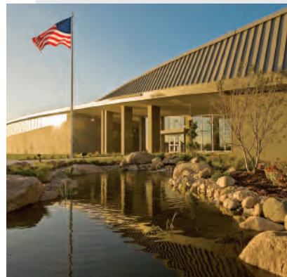
Platte West Water Treatment Plant
