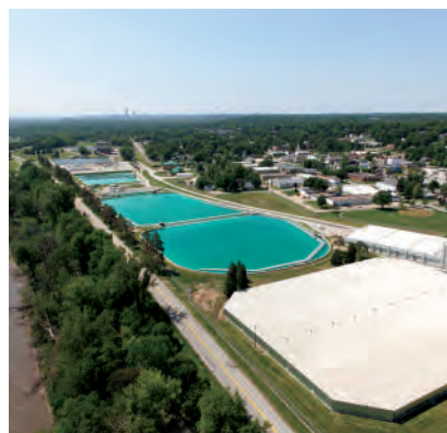
Florence Water Treatment Plant
