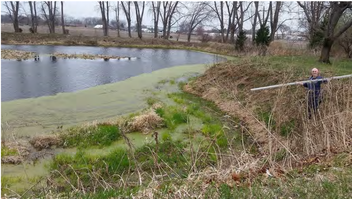
Photograph 1: View of DG-17 looking east, March 23, 2016.
