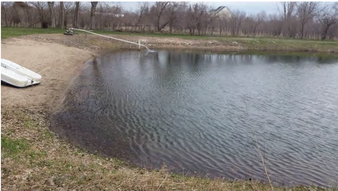
Photograph 4: View of DG-11 looking north, March 23, 2016.
