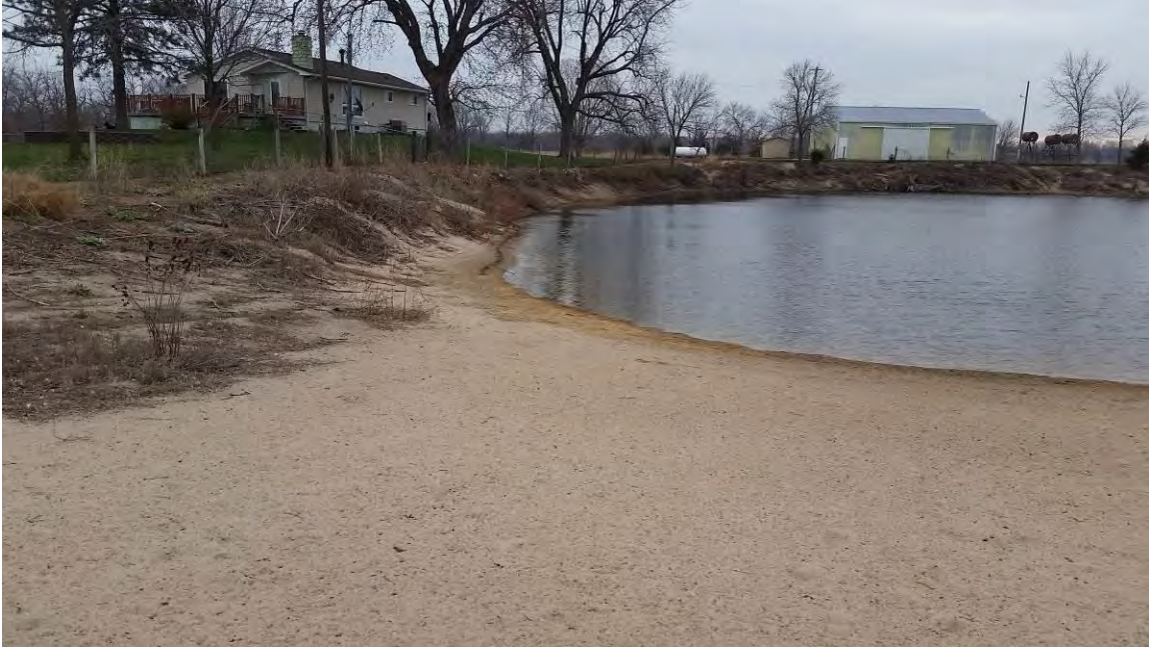
Photograph 1: View of DG-04B looking southeast, March 23, 2016.
