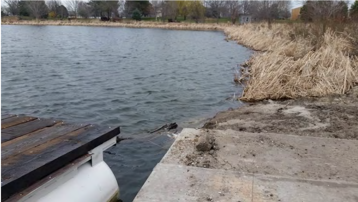
Photograph 3: View of DG-09 looking east, March 23, 2016.
