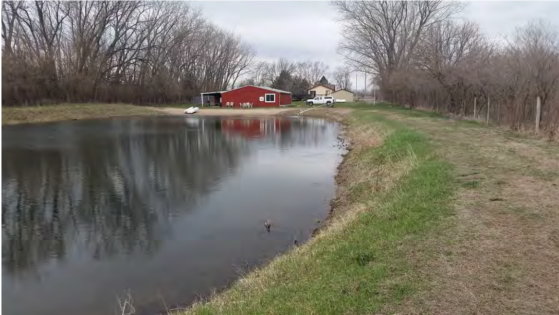
Photograph 3: View of DG-11 looking west, March 23, 2016.
