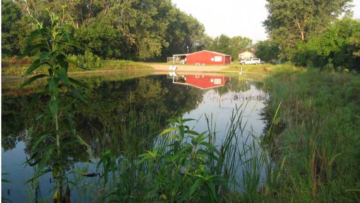
Photograph 7: View of DG-11 looking west, August 18, 2016.
