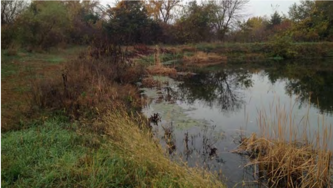
Photograph 13: View of DG-11 looking south, October 20, 2016.
