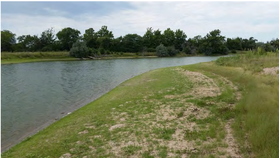
Photograph 6: View of DG-52 looking northwest, August 18, 2016.
