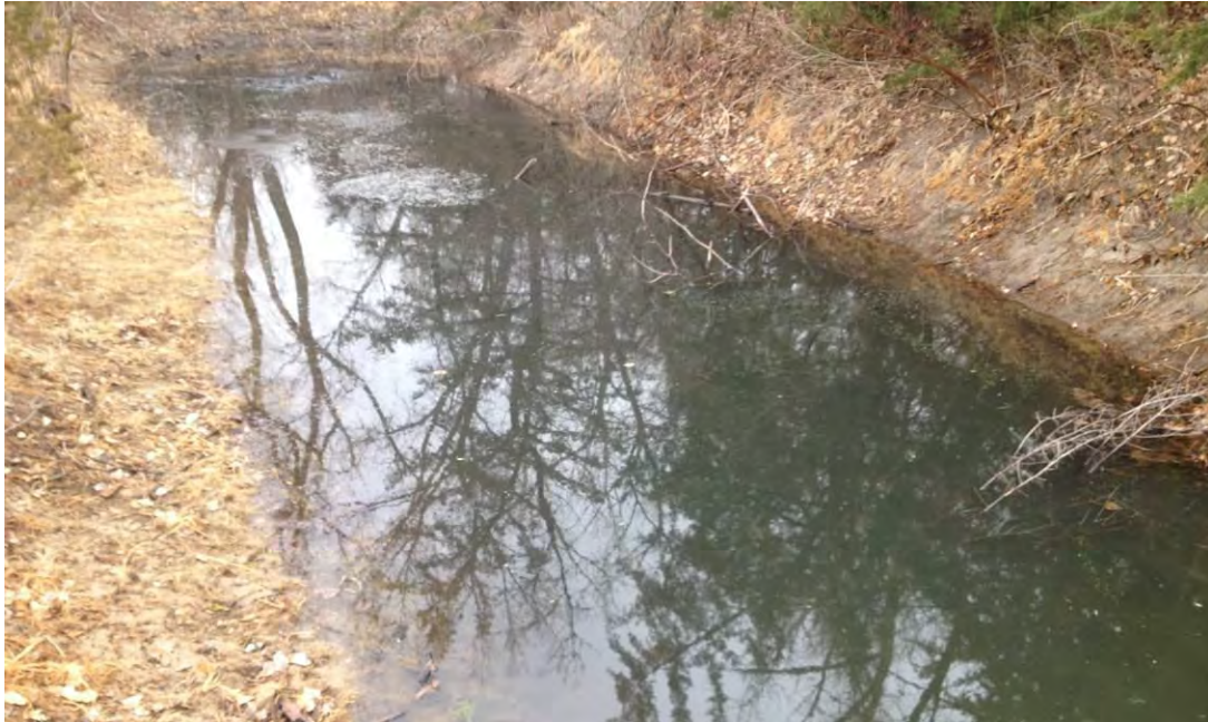
Photograph 1: View of DG-20E looking southeast, March 23, 2016.
