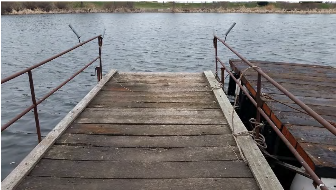
Photograph 2: View of DG-09 looking north, March 23, 2016.
