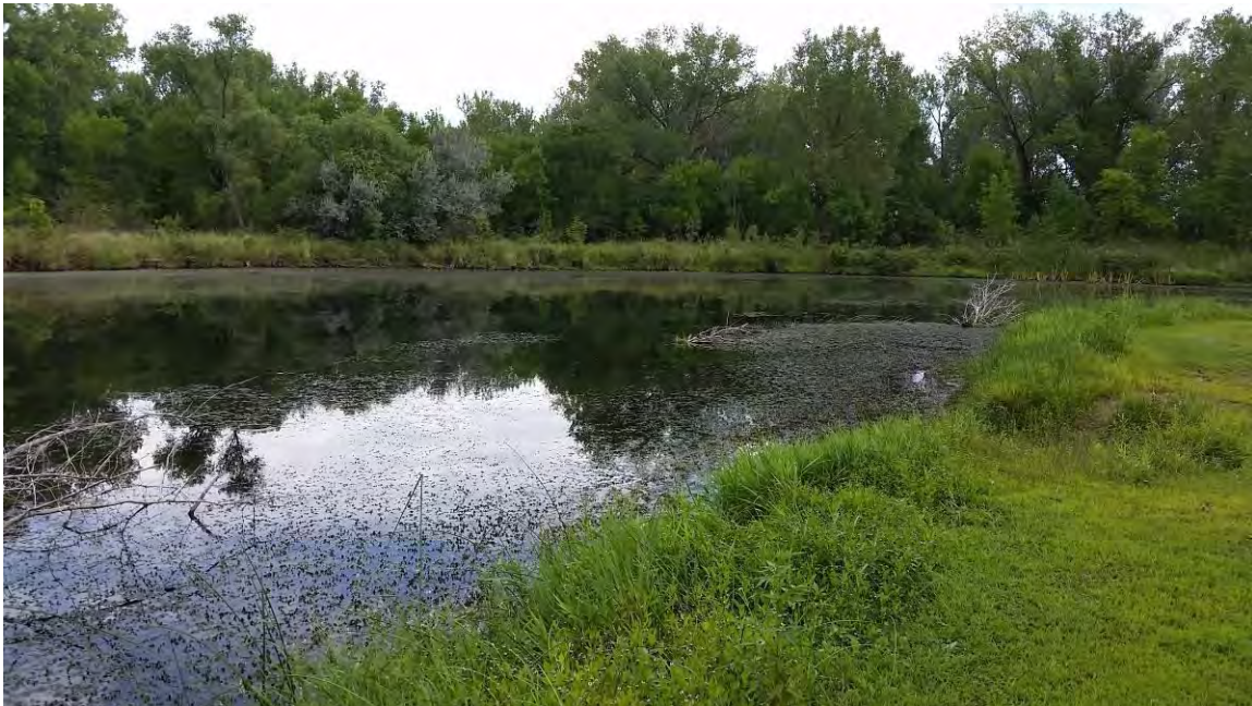
Photograph 4: View of DG-26 looking northeast, August 18, 2016.
