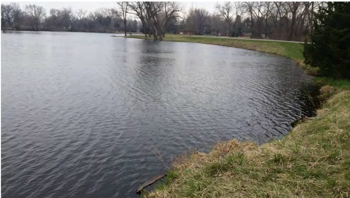
Photograph 2: View of DG-29 looking southeast, March 23, 2016.
