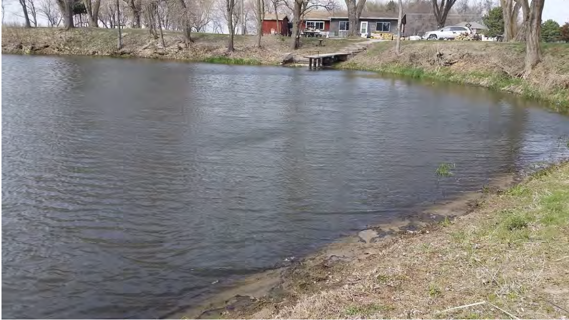
Photograph 3: View of SN-16 looking northwest, March 23, 2016.
