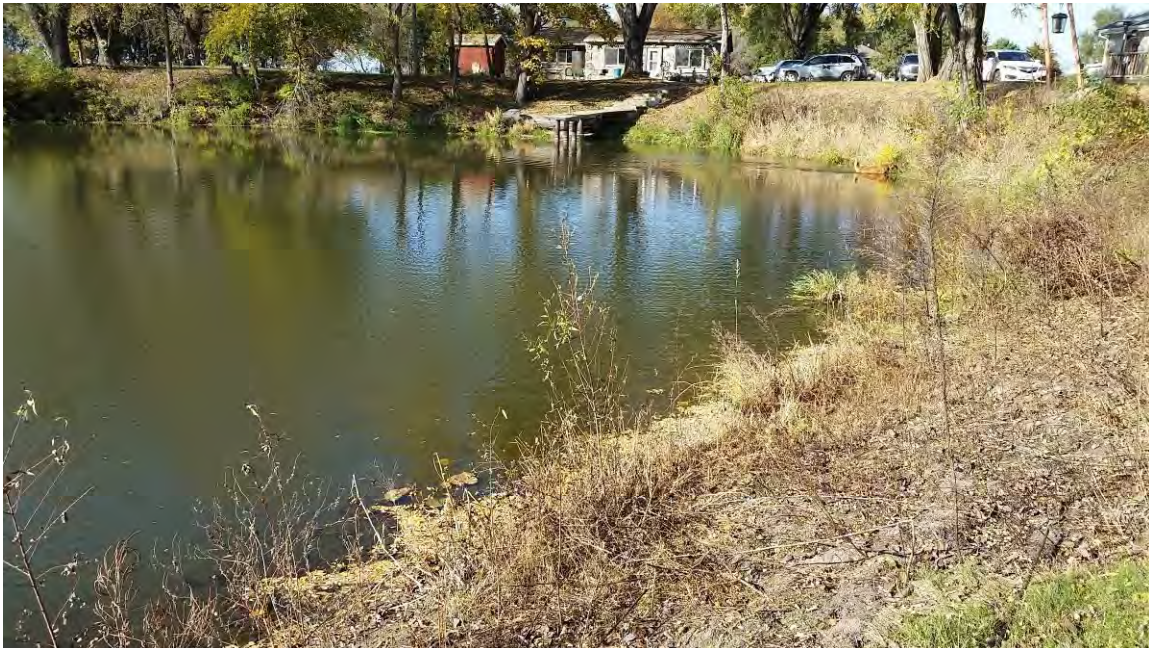
Photograph 12: View of SN-16 looking northwest, October 20, 2016.
