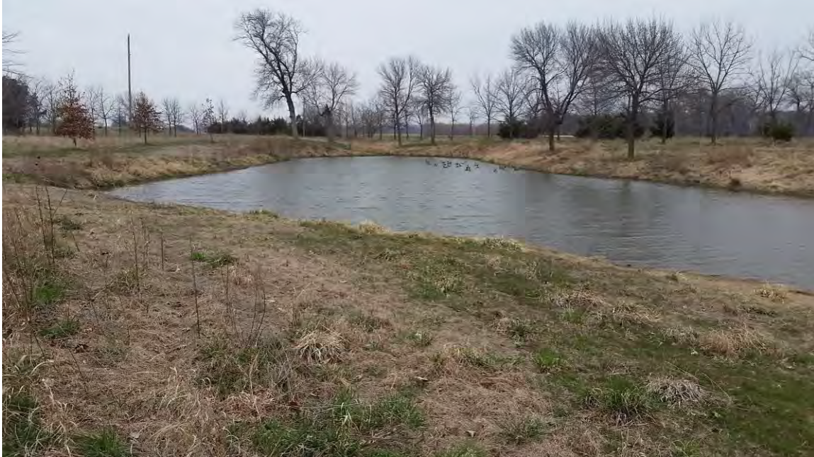
Photograph 1: View of DG-04A looking northeast, March 23, 2016.
