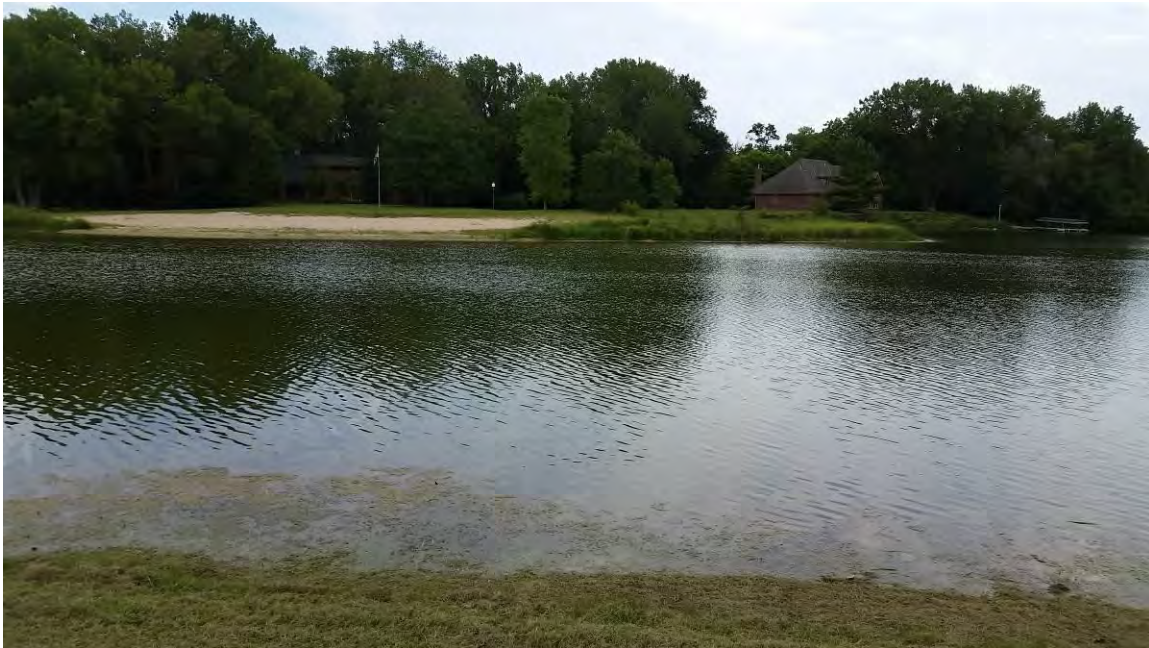
Photograph 4: View of DG-46 looking southeast, August 18, 2016.
