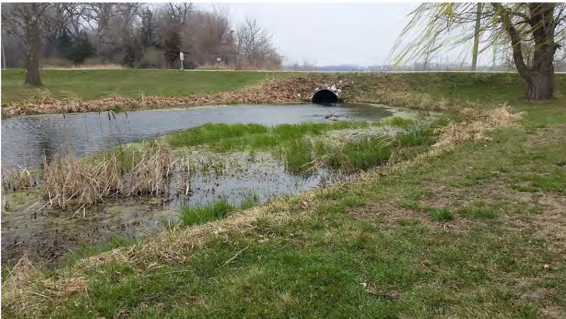
Photograph 2: View of DG-32 looking northwest, March 23, 2016.
