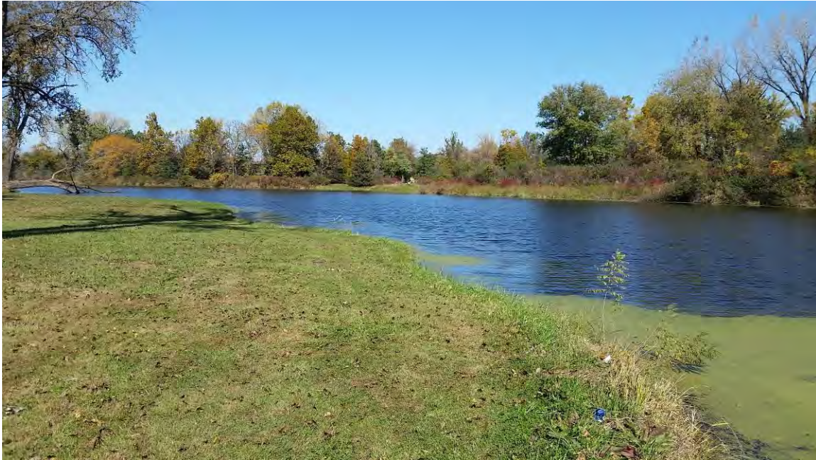
Photograph 7: View of DG-30 looking north, October 20, 2016.
