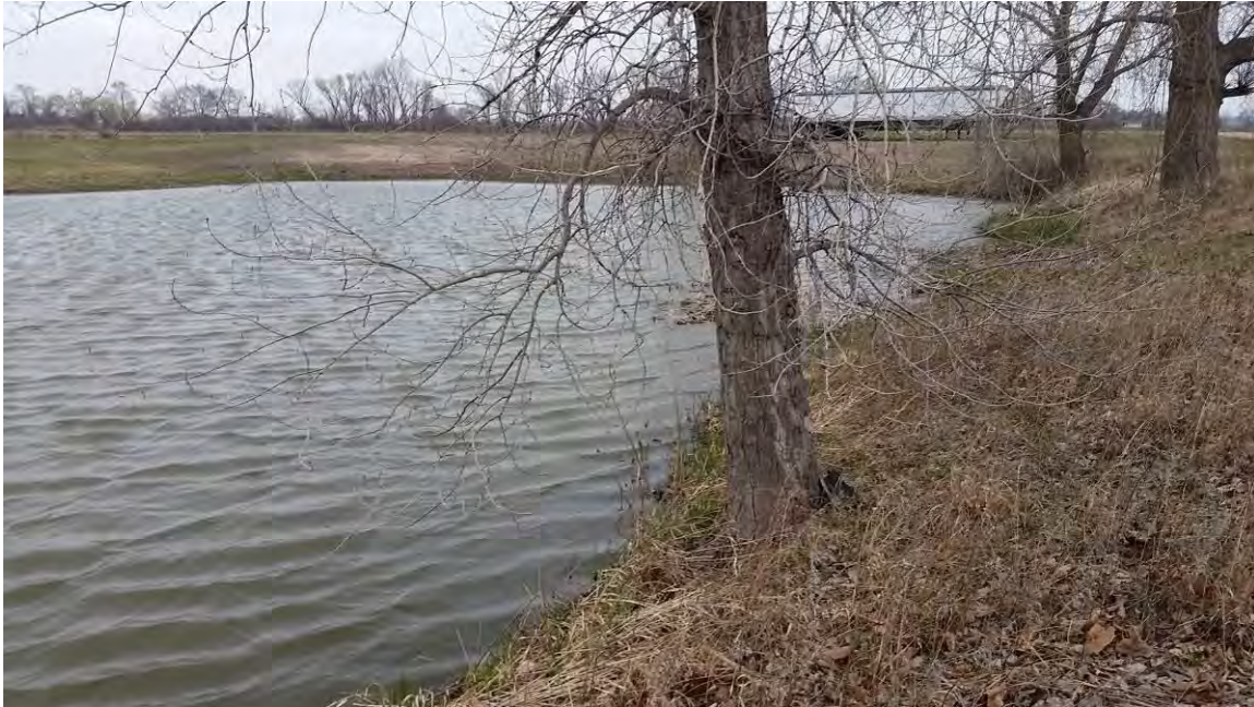
Photograph 1: View of DG-34 looking east, March 23, 2016.
