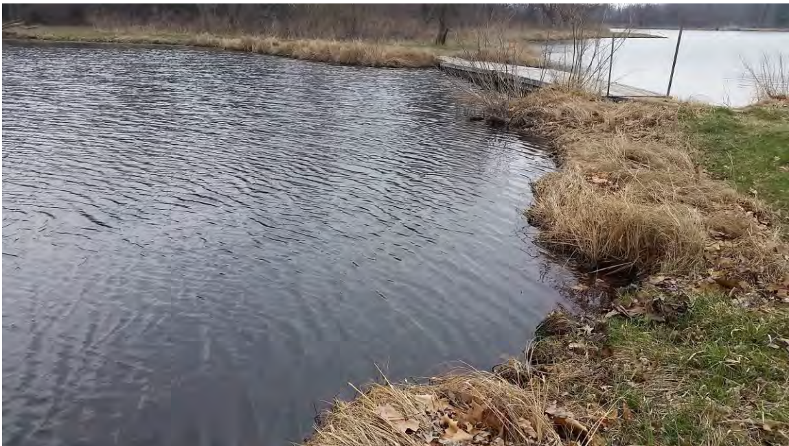
Photograph 2: View of DG-30 looking southeast, March 23, 2016.
