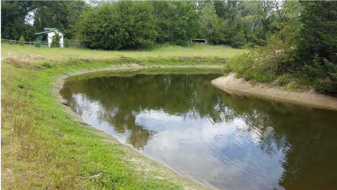
Photograph 3: View of DG-20 looking west, August 18, 2016.
