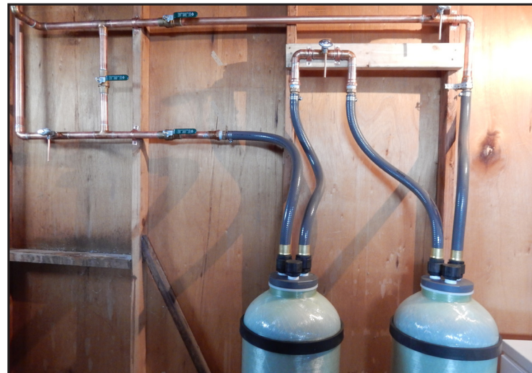
Granular Activated Carbon Unit
