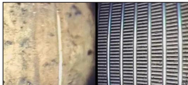
Extraction Well Screen Before and After Cleaning with Sonar Jet™
