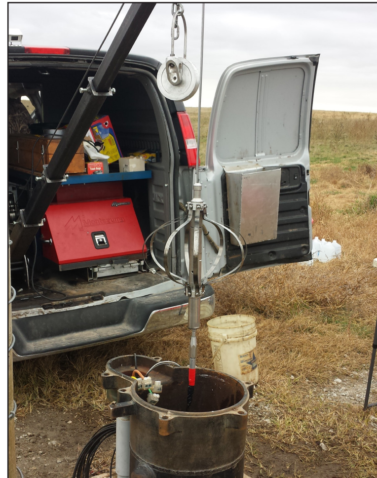
Sonar Jet™ Cleaning Device Being Lowered into an Extraction Well
