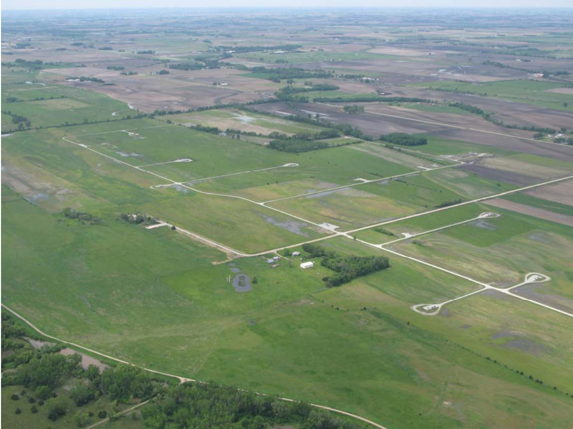
Wellfield Construction (Taken June 1, 2008) Aerial View Looking Southwest – Saunders County Wellfield
