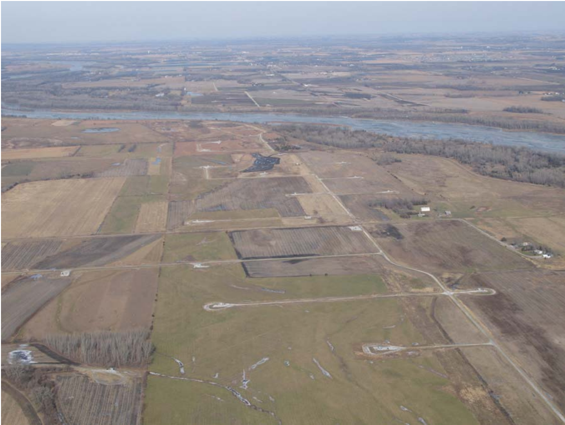
Wellfield Construction (Taken December 3, 2007) Aerial View Looking North – Saunders County Wellfield
