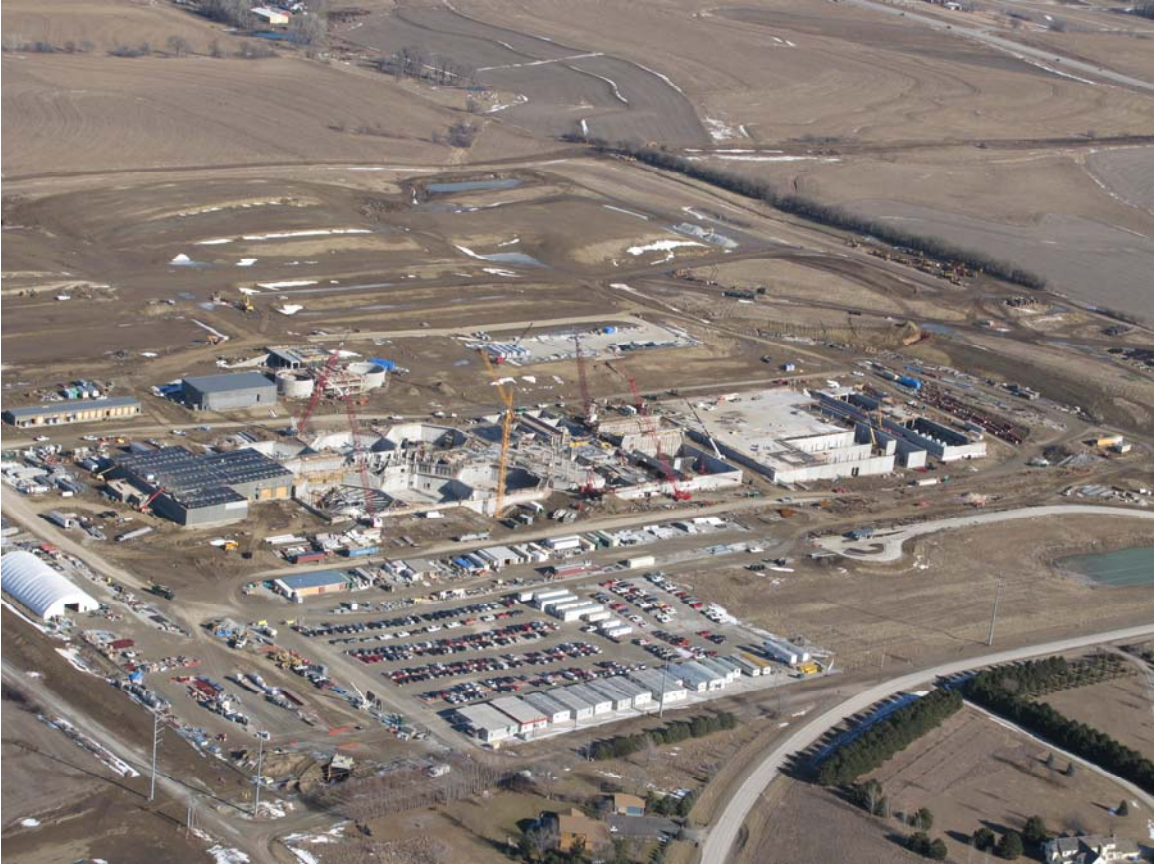
Water Treatment Plant (Taken January 8, 2007) Aerial View Looking Northeast (Intersection of 216 th and Q Streets in lower left corner)
