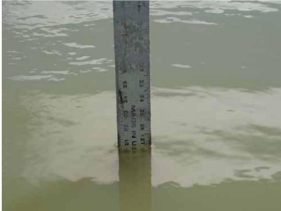
Photograph 7: View of DG-15 staff gauge, September 18, 2006.
