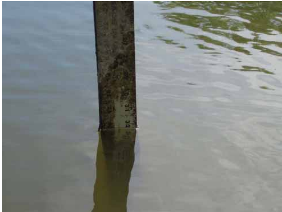
Photograph 4: View of DG-13 high water staff gauge, August 15, 2006.
