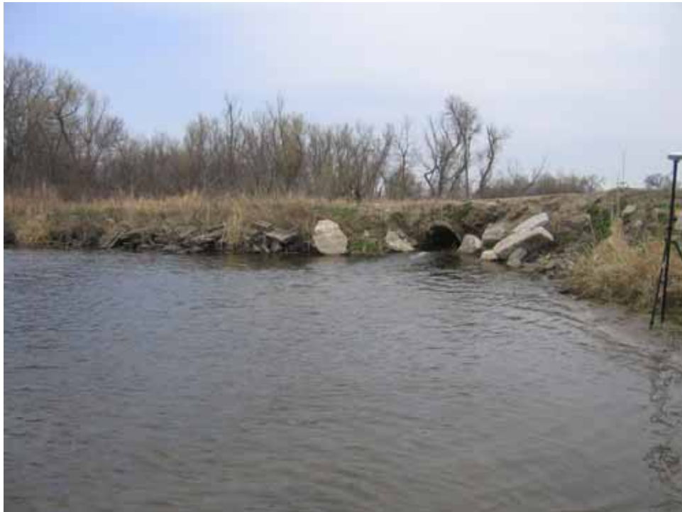
Photograph 6: View of DG-02 looking north, April 5, 2006.
