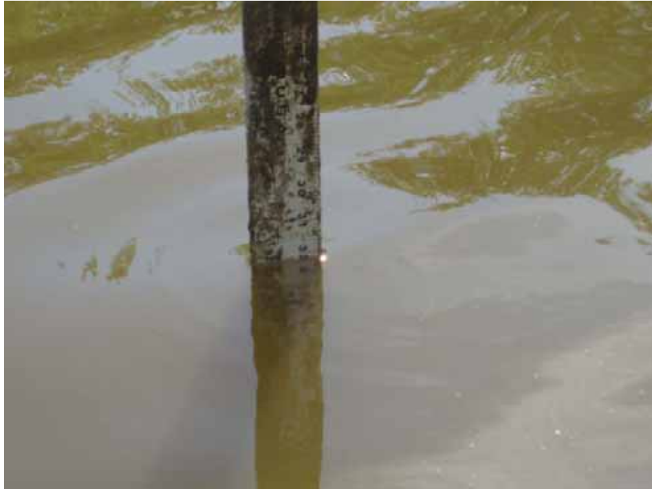
Photograph 7: View of DG-02 staff gauge, August 15, 2006.
