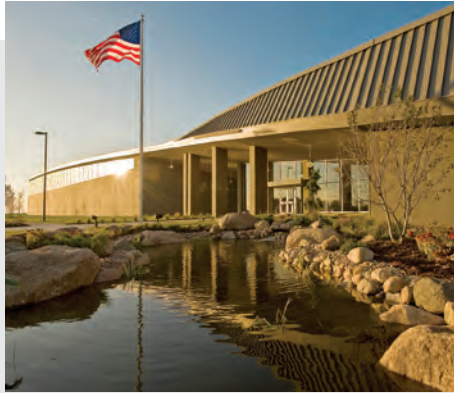
Platte West Water Treatment Plant
