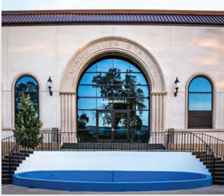
Florence Water Treatment Plant
