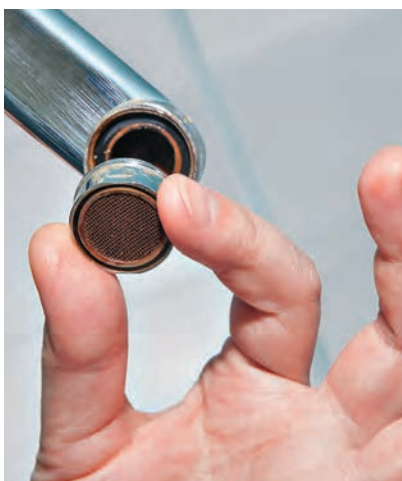
Remove and clean faucet aerators (screens) on a regular basis.
