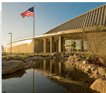
Platte West Water Treatment Plant
