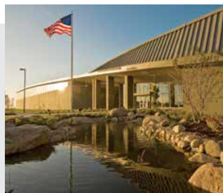
Platte West Water Treatment Plant
