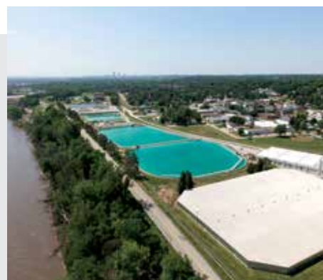
Florence Water Treatment Plant
