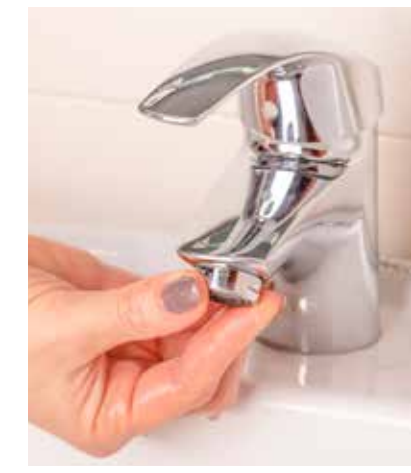
Remove and clean faucet aerators (screens) on a regular basis.
